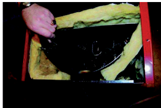
Fig 2 Pull out all turbulators.
